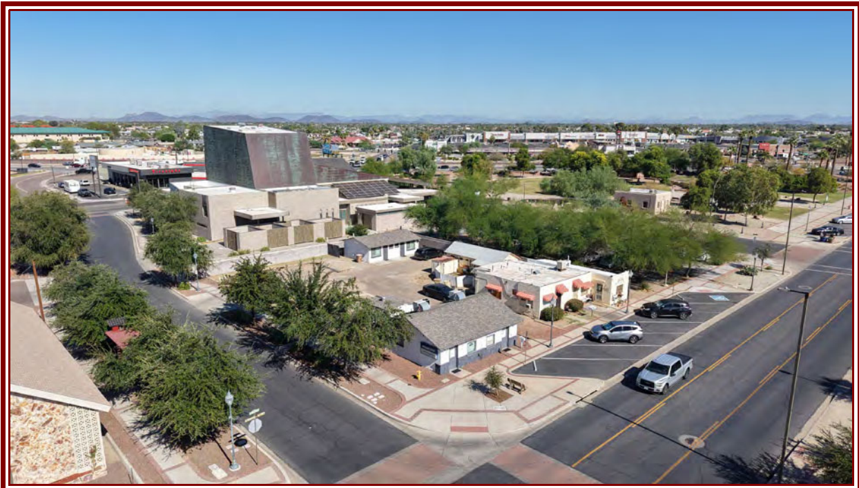
Northeast View Across The Intersection Of Washington Street And 84 th Avenue The Subject Property Wraps Around The Northeast Corner Of Intersection
