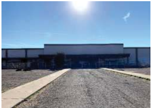
12. Former Smitty's building
