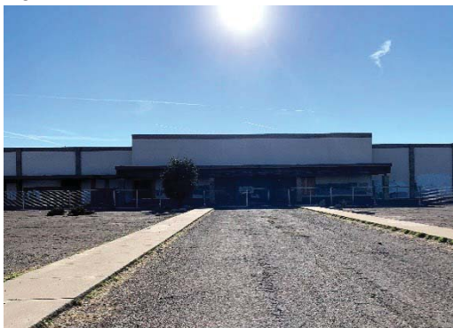
12. Former Smitty's building
