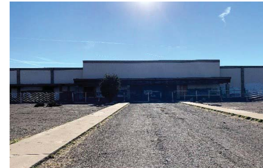
12. Former Smitty's building
